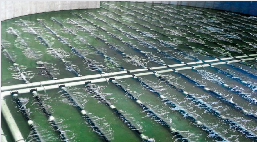
Tubular System Diffusers
